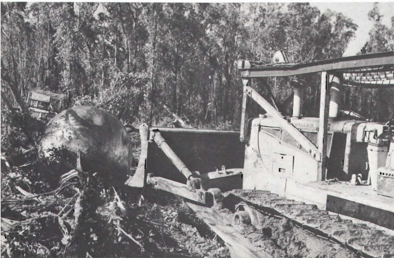
Clearing operations at Heytesbury showing a ball and chain.
